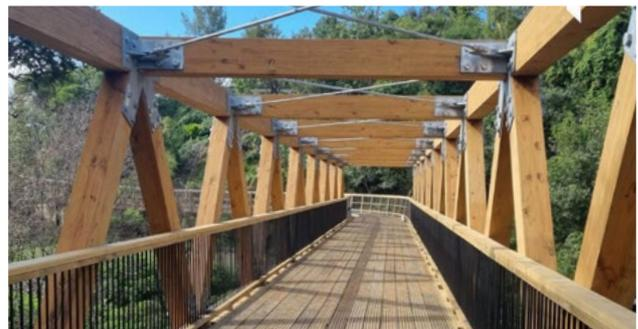
Timber Structure Bracing
