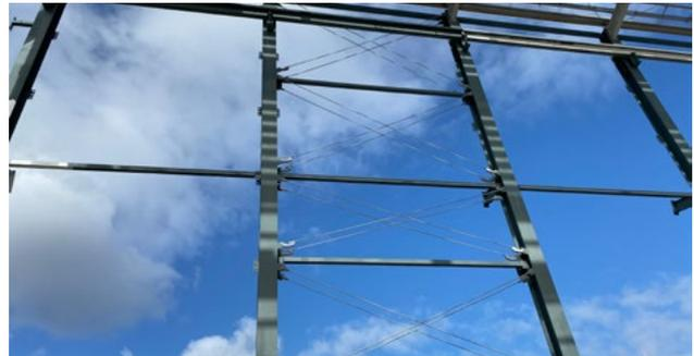
Structural Steel Structure Bracing
