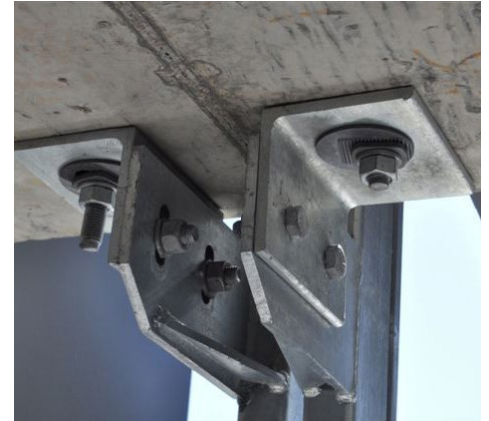
Upper connection: Reid OrbiPlate and Ramset TruBolts
