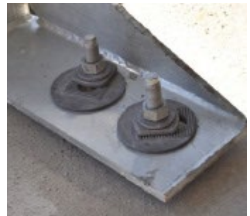
Lower Connection: Reid OrbiPlate and Ramset ChemSet 502
