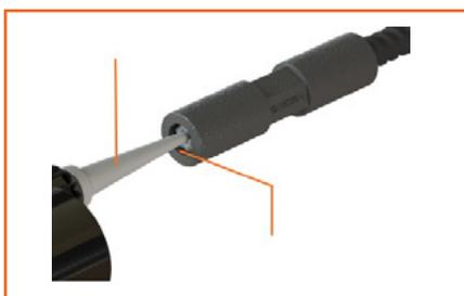
5. Screw in the second ReidBar™ into the steel coupler, and tighten the bar using a wrench to ensure that the ReidBar™ is hard against the stop. Wipe excess filler with cloth/fabric/carton as applicable.
