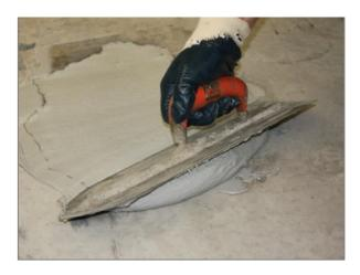
Ramset Epoxy Paste 1210 is a tough, trowellable epoxy repair mortar for use in high build concrete repair applications.
